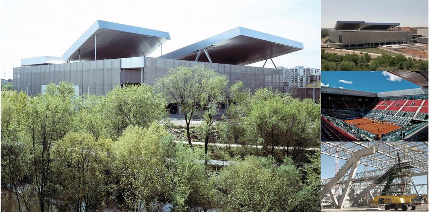
The roof of the Magic Box covers an area of three stadiums. The main stadium has a seating capacity of approximately 15,000 spectators, while the smaller stadiums 2 and 3, seat 3,000 and 4,000 people, respectively. Its large dimensions of 170.40 x 163.20m<sup>2</sup>, convert it into a significant architectural element, particularly because of its three mobile roofs.
